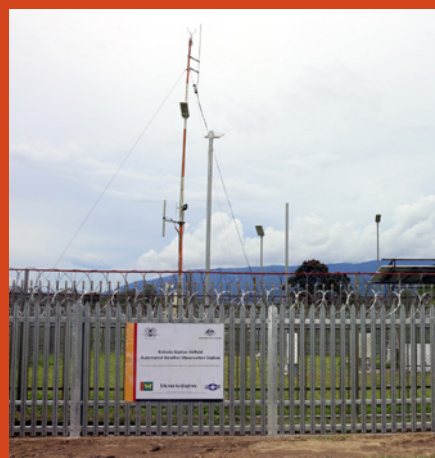
Kokoda Automatic Weather Observation Station with new security fencing and lights
